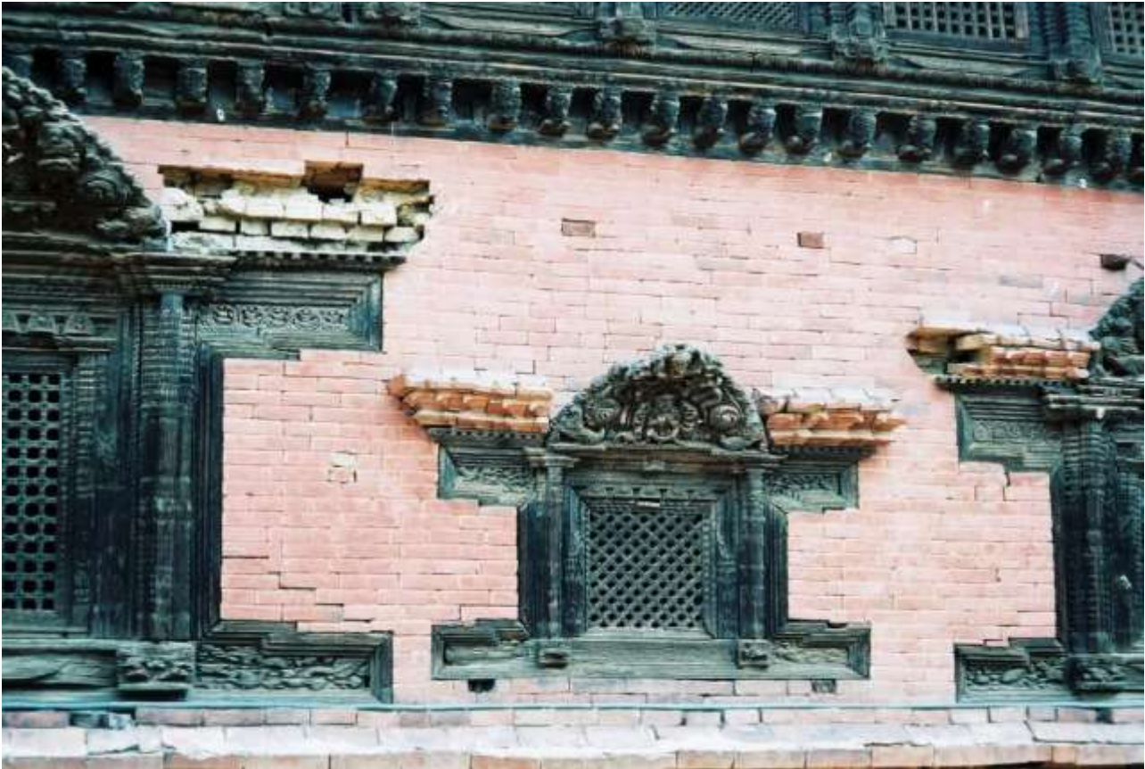
55 Windows Palace in Bhaktapur prior to 2005 restoration.
