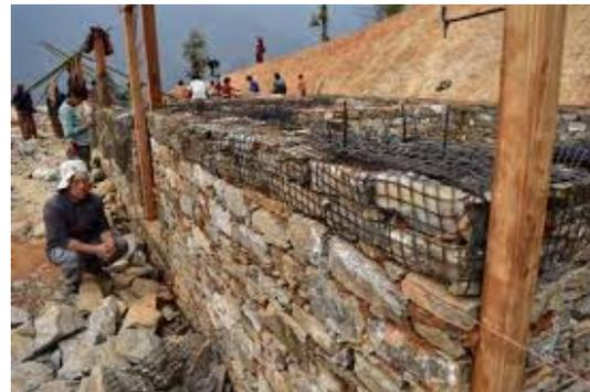
*Rebuilding rural stone houses in earthquake zones with gabion bands*
