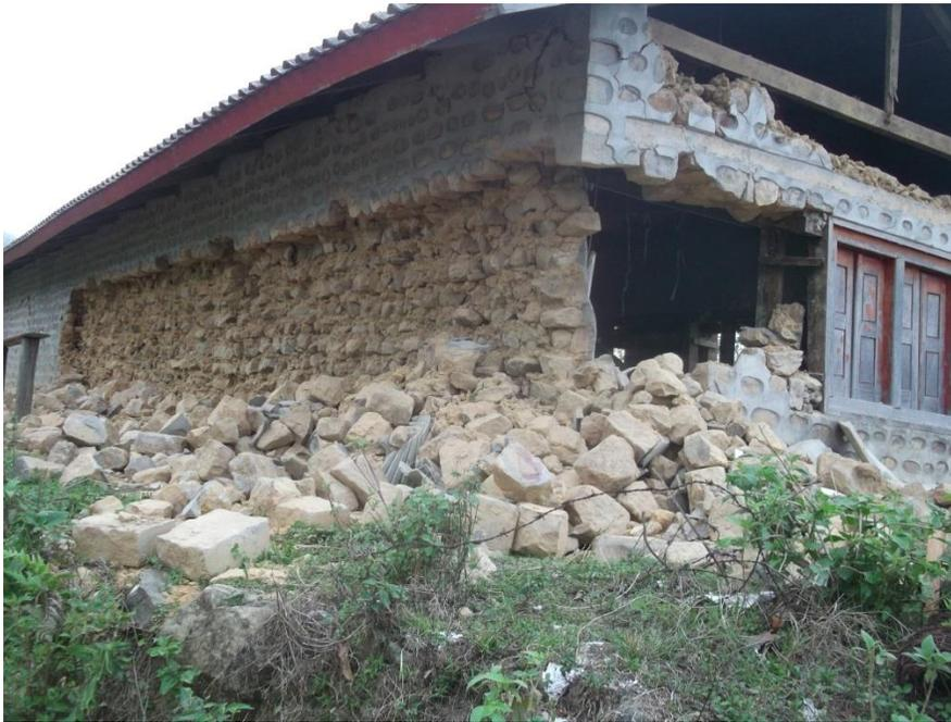
**School building in Banakhu, Kavre District showing stone fallen out from beneath RC band. The building was destroyed, and subsequently demolished. Photo by: Jeet Bahadur, Banakhu**
