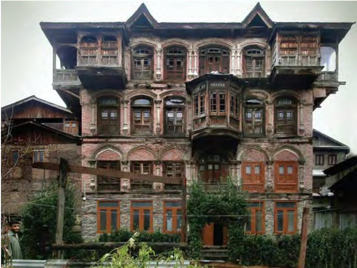
3.6.3c The Gargoo Residence in Bulbul Lankar, Ali Kadal, Srinagar. This house is four storeys plus attic in taq construction, with a stone base and brick upper storeys. Photo by Akshay Kaul.
