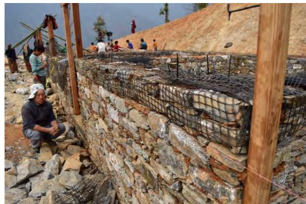
Chupar School under construction with polypropylene Gabion Bands. (Photos by John Vavruska)
