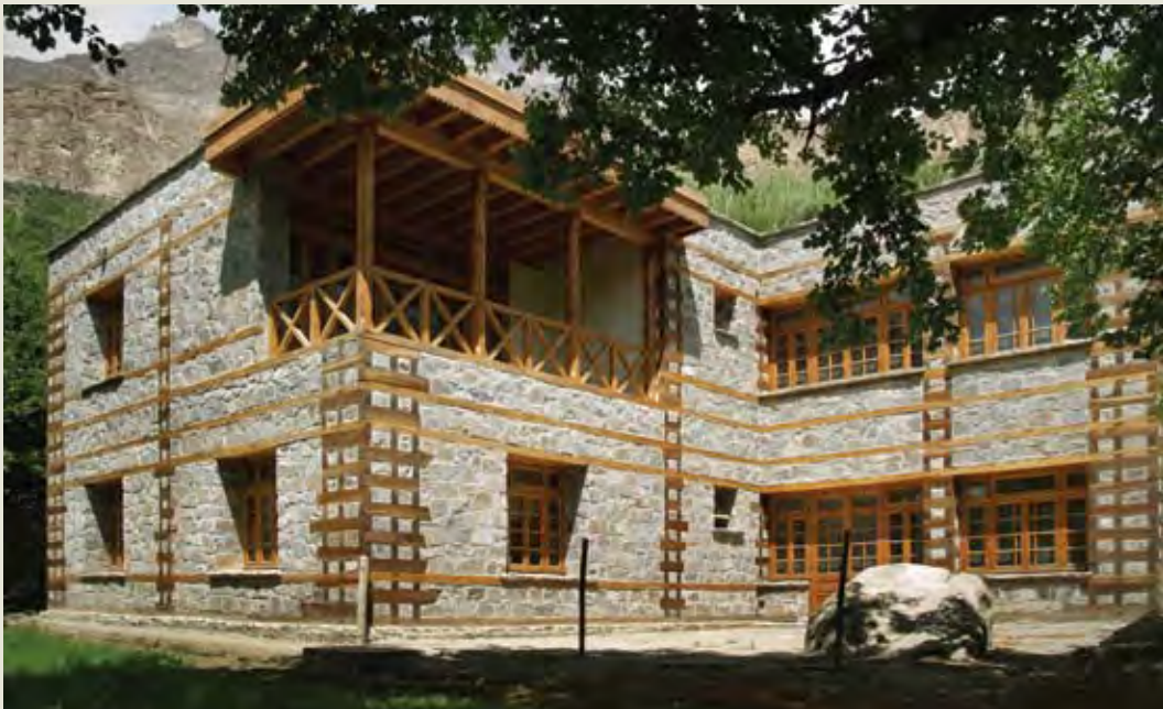
5.5h A new house with cator and cribbage timber lacing. The Balti word cator has the same meaning as the Pashto word bhatar. The regional difference is to have the extra reinforcement provided by the cribbage in the corners. This house was constructed for the former owner of the historic Altit Fort by the Aga Khan Cultural Services Division. Photograph by Tom Schacher, Swiss Agency for Development and Cooperation (SDC).
