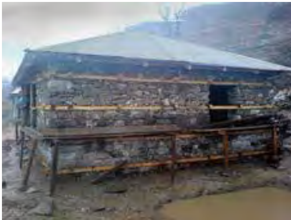
left: House in Pakistan of bhatar construction being built after 2005 earthquake (photo by Tom Schacher for SDC). Right: Demonstration house with Gabion Bands at the Sunar Family Farm in Mankhu, Dhading District featured in TV documentary show Himalayan Megaquake.
