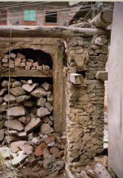
1.1e Photograph taken in the 1980s showing a building under demolition with taq timbers visible at the window lintel level and at the floor level. The floor joist can be seen to penetrate the wall where it is sandwiched between the exterior runner beams.
