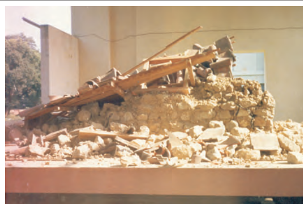
Fig. 10 Unstrengthened house constructed with mud mortar
