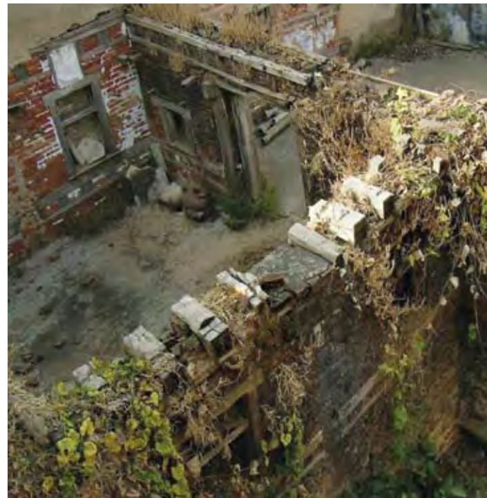
1.1h View of partially demolished 18th- or 19th-century dwelling in Ahmedabad, Gujarat, with timber lacing like that found in Kashmir. This view shows the cross-pieces that tie the inside and outside runner beams laid into the masonry wall together. (A view of the peg holding one of these crosspieces is shown in Figure 2.3.3a.)
