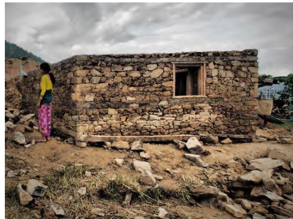
left: House in Pakistan of bhatar construction being built after 2005 earthquake (photo by Tom Schacher for SDC). Right: Demonstration house with Gabion Bands at the Sunar Family Farm in Mankhu, Dhading District featured in TV documentary show Himalayan Megaquake.
