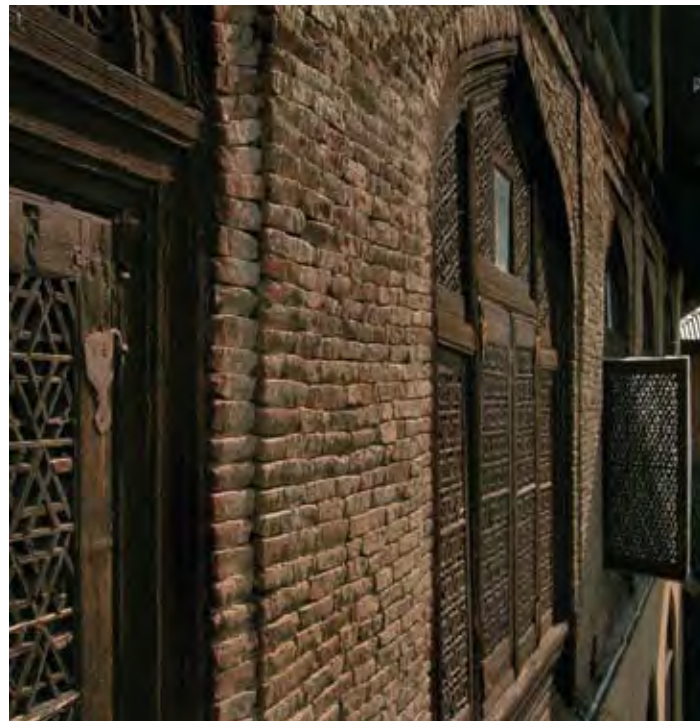
1.1f View of the mid-19th century Jalali Haveli in Srinagar showing Maharaji bricks. Maharaji bricks, common in the 18th to early 20th centuries, were shaped without the use of a wooden mold and thus are of varying length and about 1 inch (2.5 cm) in thickness.
