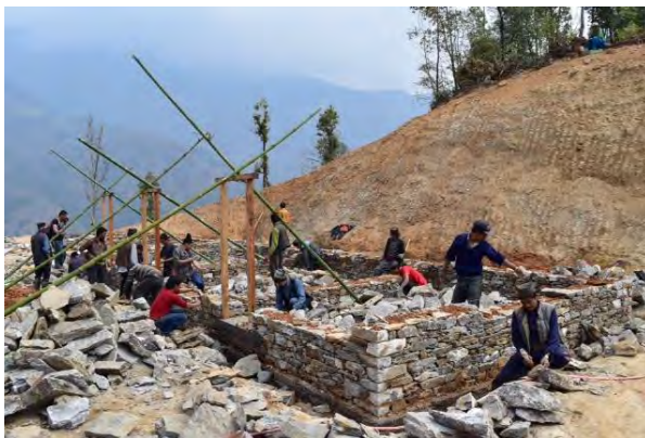
Chupar School under construction with polypropylene Gabion Bands. (Photos by John Vavruska)
