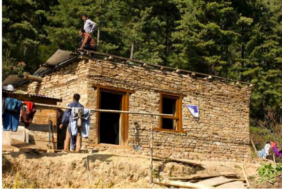
New house with Gabion Bands in Jiri.
