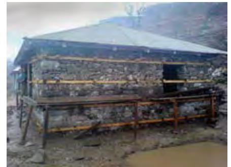
3.3i & j Completed building with bhatar following the Pakistani government-endorsed guidelines constructed by SDC as a demonstration of approved bhatar detailing. Photos by Tom Schacher, SDC.
