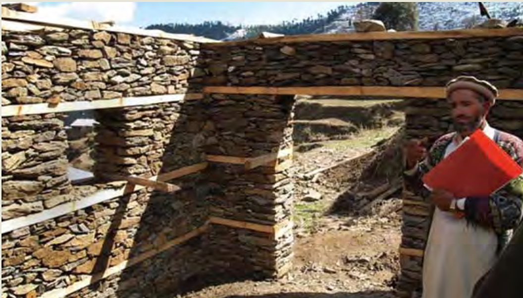
5.5i This new barn of bhatar with dry-laid stone masonry construction is in a mountain village near Battagram (in Gari Nuwab Said) in the Northwest Frontier Province of Pakistan. The site is remote from the road, one hour by car, then another half-hour by foot away from Battagram, making reinforced concrete construction impossible. Photograph taken in 2007 by Tom Schacher, Swiss Agency for Development and Cooperation (SDC).
