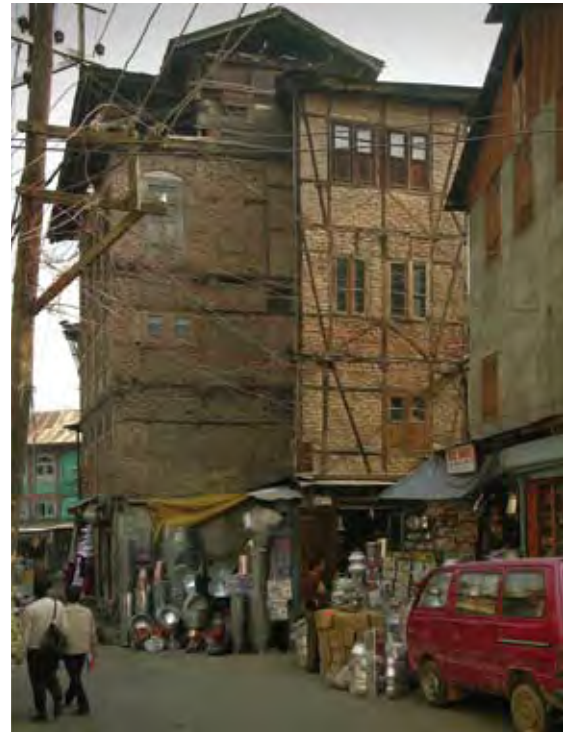
3.6.3b A five-storey (including attic level) taq building and four-storey dhajji dewari building in the commercial centre of Srinagar. These and many others in Srinagar may be reminiscent of the kinds of buildings which astonished Kalhana in 1148, Tímúr in 1398 and Dughlat in 1540.
