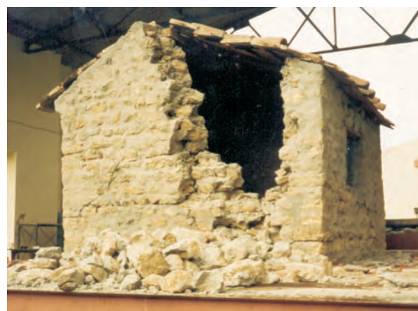
Fig. 9 Unstrengthened house of cement-sand mortar
