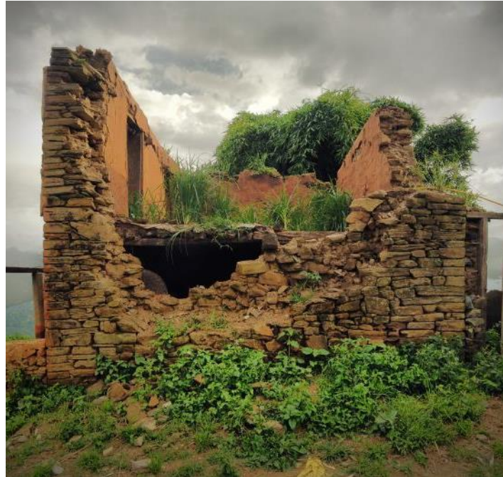
The above photos show the ruins of the main house at the Sunar Farm. This wall shows evidence that the collapse of the wall resulted from the separation of the inside and outside leafs and the spreading of the stones at the corners.
