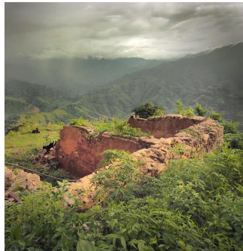
A view of the ruin in the site of the demonstration house on the Sunar Farm, in Mankhu. This was photographed the day before work was started at the site. The construction process to the point shown on page 7 was completed in four days.
