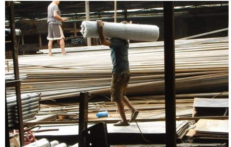
Above shows a roll of wire mesh for Gabion Bands being carried. Only about 2.5 rolls were needed for the house shown in this report. This can be compared with carrying of cement, sand and rebar for concrete, as is shown below. (Photos by Randolph Langenbach)
